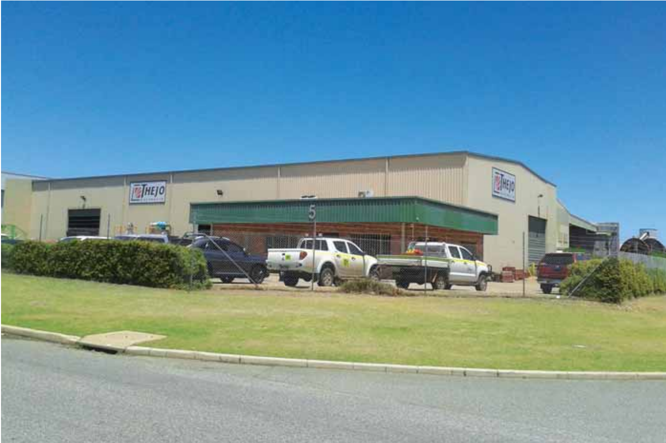
Perth Office of Thejo Australia Pty Ltd.
