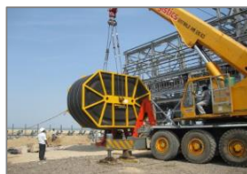
Conveyor belt laying (Conveyorbelts)
