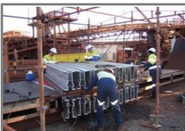
Conveyor belt splicing service (Steel cord belts, fabricply belts)
