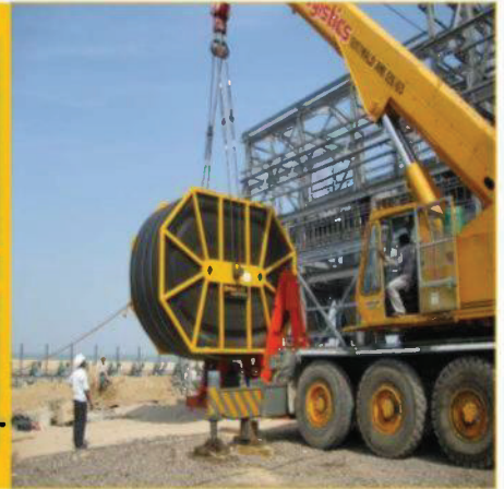
Comprehensive Operation & Maintenance
