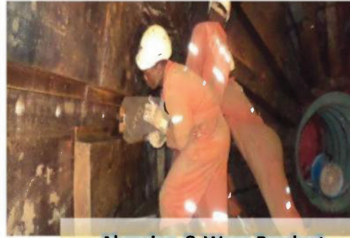
Abrasion & Wear Product Installation
