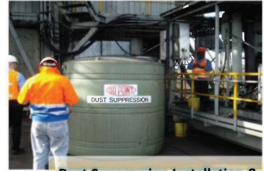
Dust Suppression Installation & Maintenance
