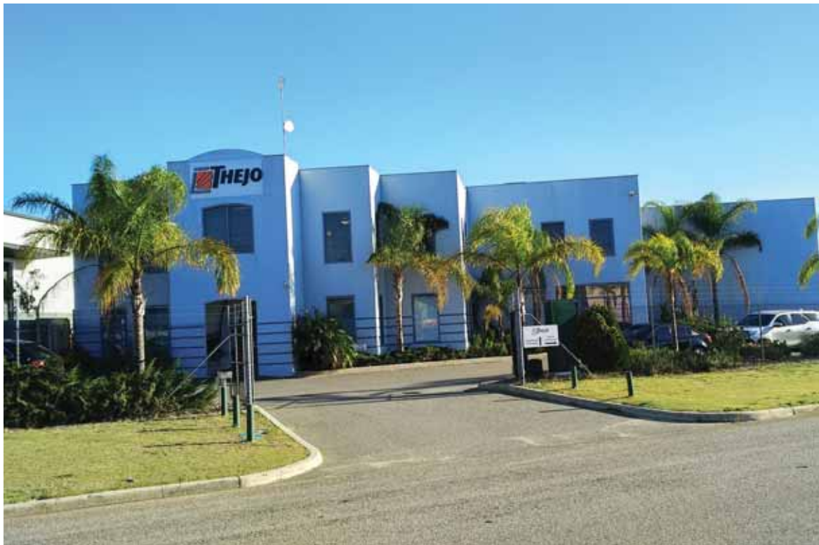
Administrative Offices of Thejo Engineering Limited and Thejo Australia Pty Ltd, Perth
