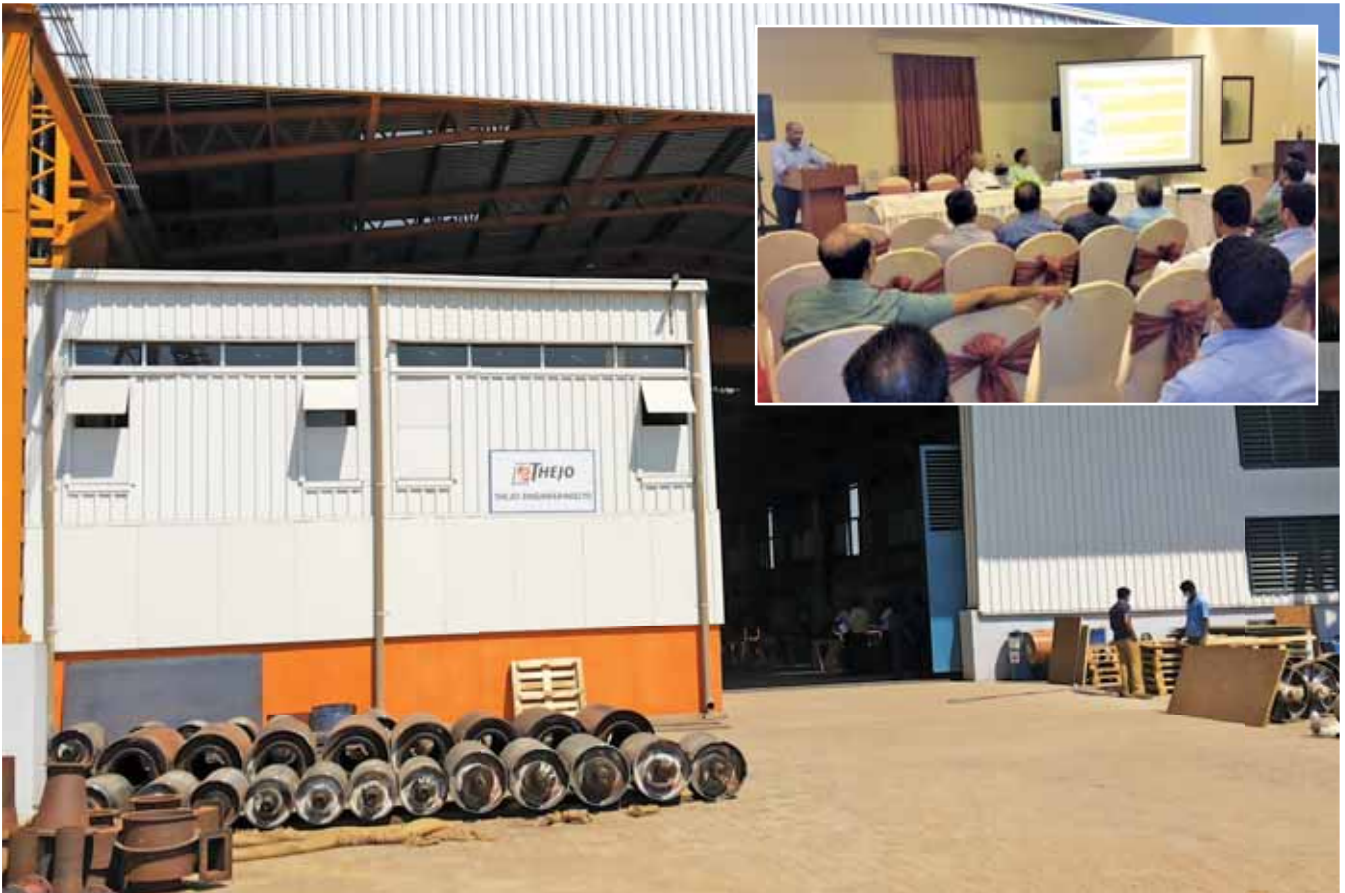
The new state of the art Lining Unit. (Inset: Clients visit & get-together during inauguration of Lining Unit.)
